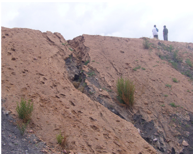
Fig. 7. Tailing after the rain
